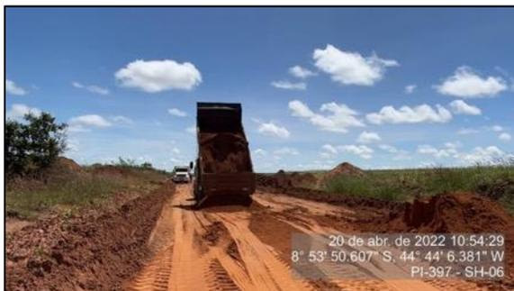
Figura 71 – Transporte e descarga – SH-06
